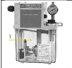
Check oil level of central lubrication before starting work or after every maintenance and repair.
